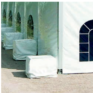
Weight anchoring by means of concrete blocks
