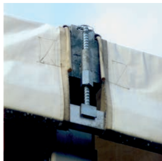
Spindle-fix roof tensioning
