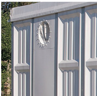
System cassette wall elements of hard-PVC with connecting panel for air conditioning and heating systems
