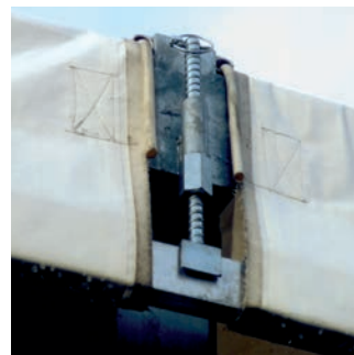
Spindle-fix roof tensioning system
